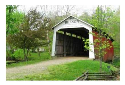
The Beeson Bridge was built in 1906 by the Frankfurt Construction Company in Marshall, Indiana, and was named for adjacent landowners. It is of Burr Arch Construction and is 55 feet long, 16 feet wide and has a clearance of 13 feet. The Beeson Covered Bridge is the only remaining bridge in Parke County built by a professional construction company. It originally crossed Roaring Creek on the back road from Marshall, Indiana.
