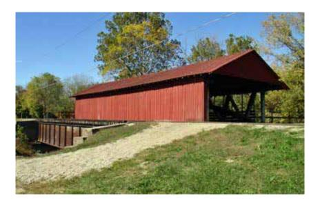
Carrying the White Water Canal across Duck Creek and constructed using a Burr arch truss, this 60-foot structure was built by Canal Trustees in 1846. The aqueduct was restored in 1946-49, and again in the 90s; another major restoration was completed in 2005. The Aqueduct is part of the White Water Canal State Memorial at Metamora and it is the only aqueduct covered bridge in the United States.
